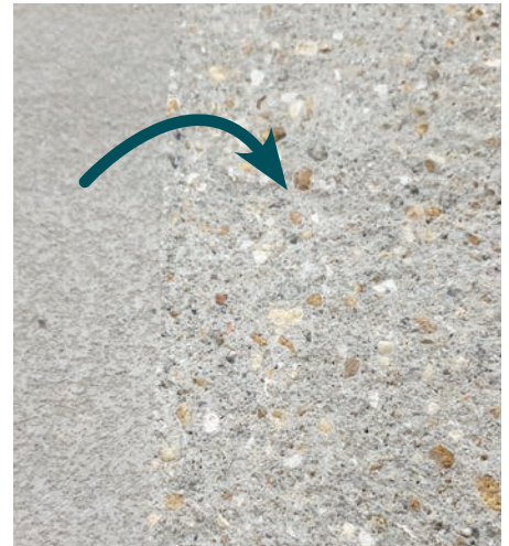
Concrete blasted, scarified, or grinded to an open texture exposed aggregate finish
